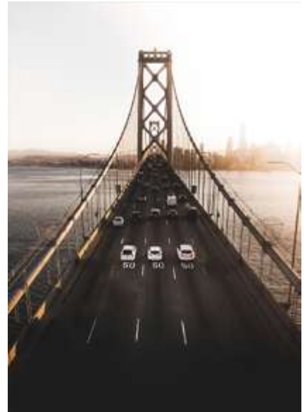
GL-12834 • GL358 • Bridge road
