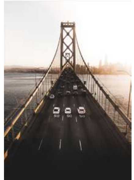
GL-12834 • GL358 • Bridge road
